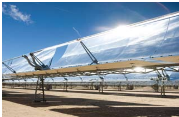
Solar power energy panels.
